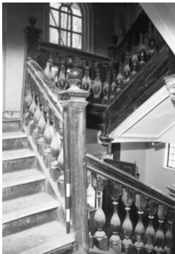
Plate 6 The ‘Talbot Stairs’ from the first landing (Building B)
