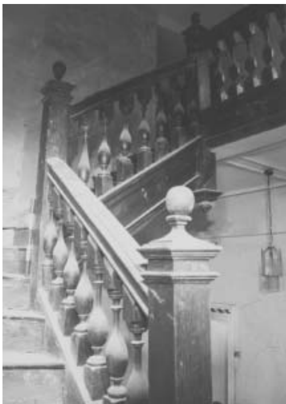
Plate 5 The ‘Talbot Stairs’ from the ground floor (Building B)
