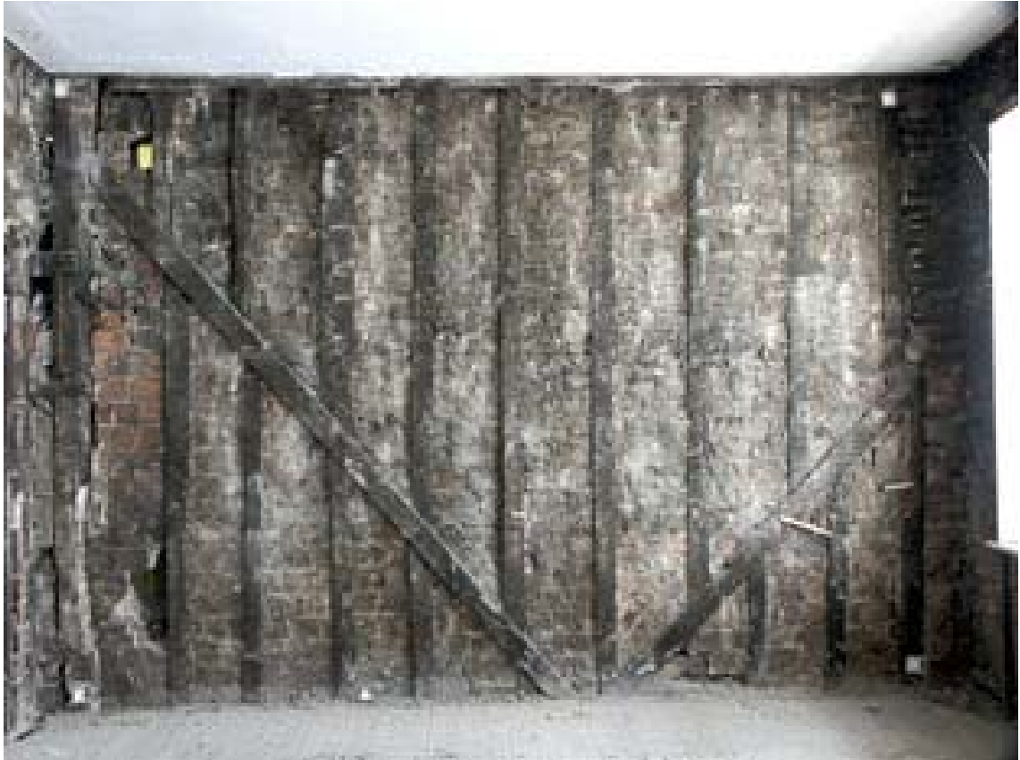
Plate 16 Internal SE wall of the SE room in Building D
