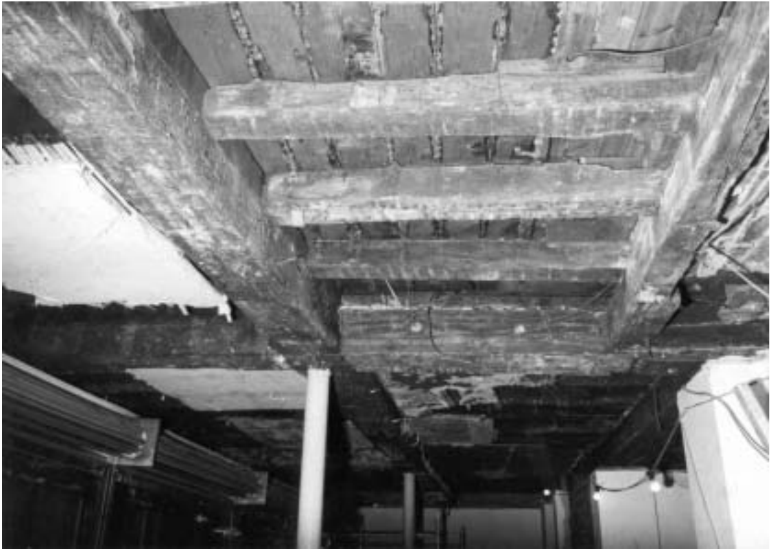
Plate 15 Ceiling on the ground floor of Building D
