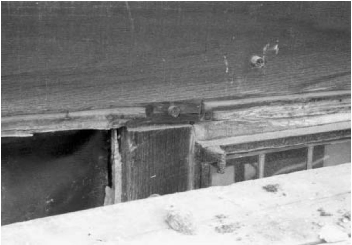
Plate 19 Moulded beam beneath the wall-plate of Building D (Elevation G1)
